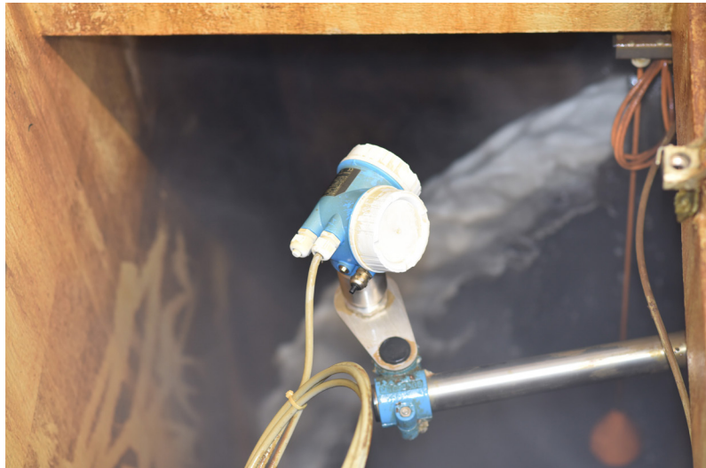
Micropilot FMR60 in the centrate water.
